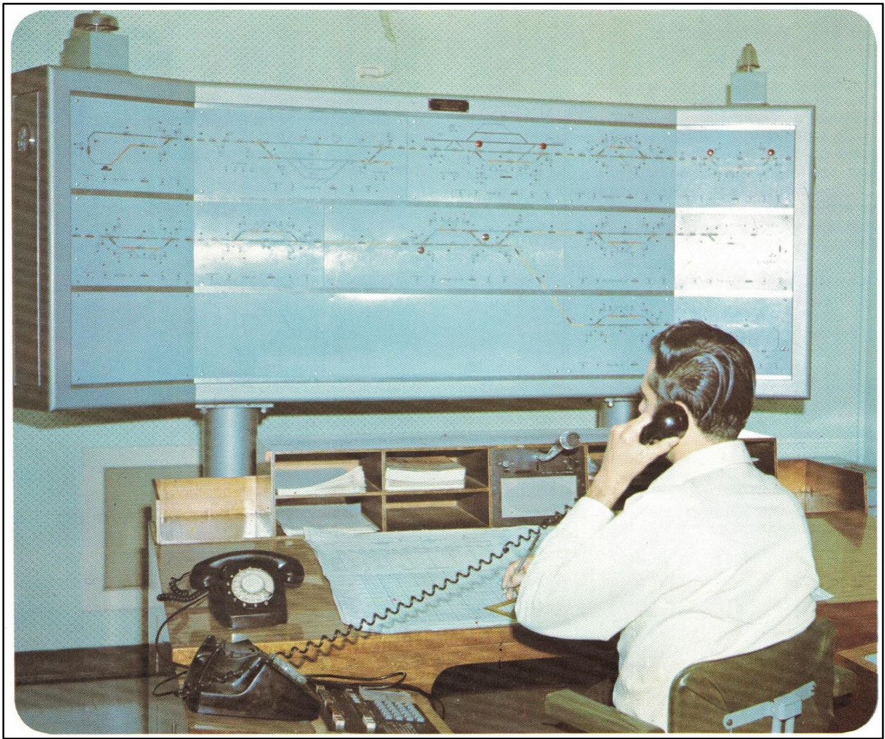
Above: The Hay Point to Goonyella and Peak Downs CTC mimic panel in the control room at Mackay. Image: QR Annual Report 30-6-1973
