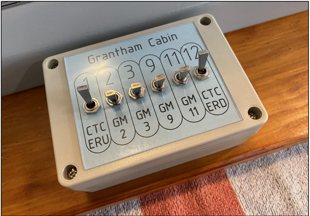
Above: The small switch box used to simulate the levers in the signal cabin controlling the signals and Electric Releases.
