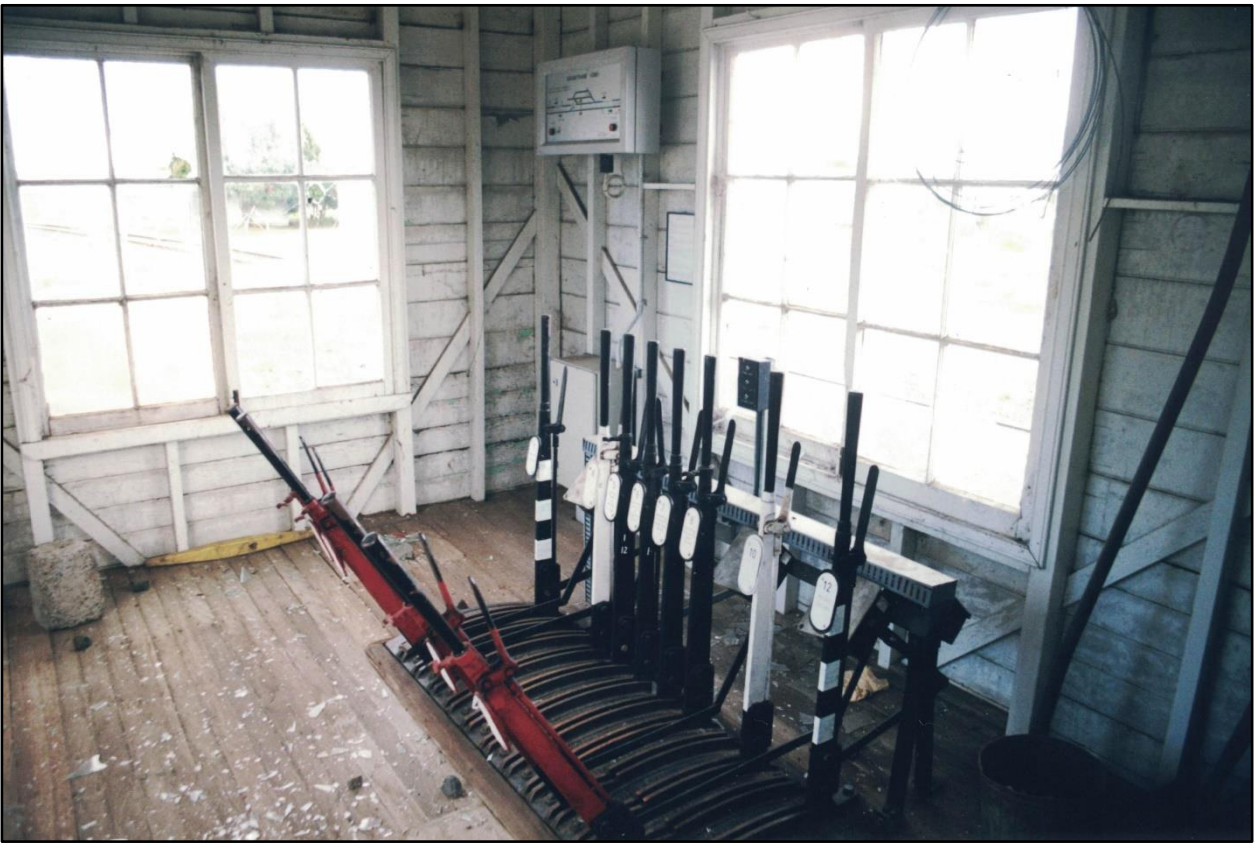
Above: Seven years after the Station Master had been abolished the building was partly vandalised and would soon be decommissioned totally. An instruction chart on the wall described the procedure to cut-in and cut-out the cabin.
