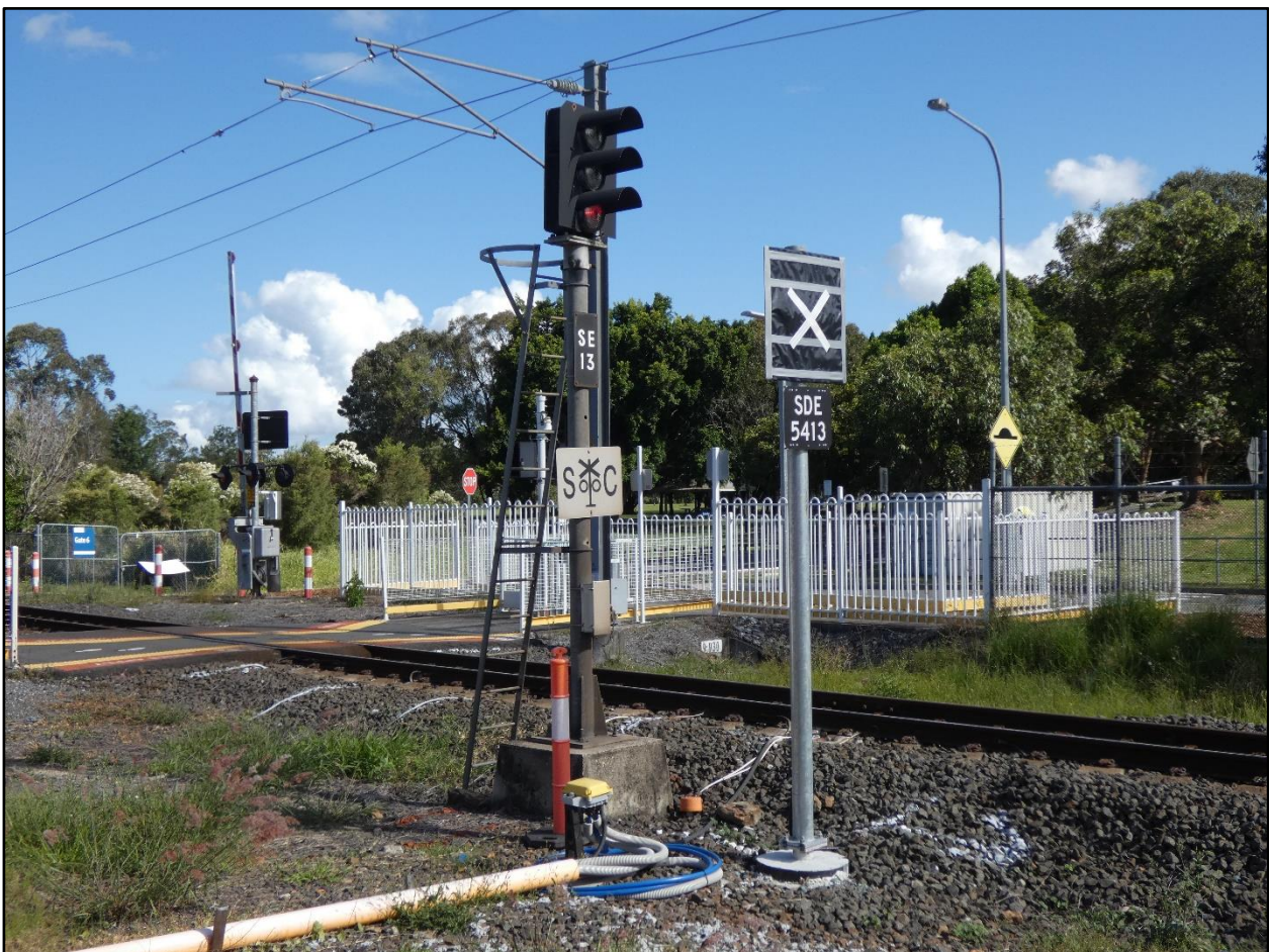
Above: Sandgate signal SE13 soon to be replaced with Block Limit Marker SDE 5413. Note that the new signs have a three-letter mnemonic and in this case, the number allocated partly matches the old signal number.
