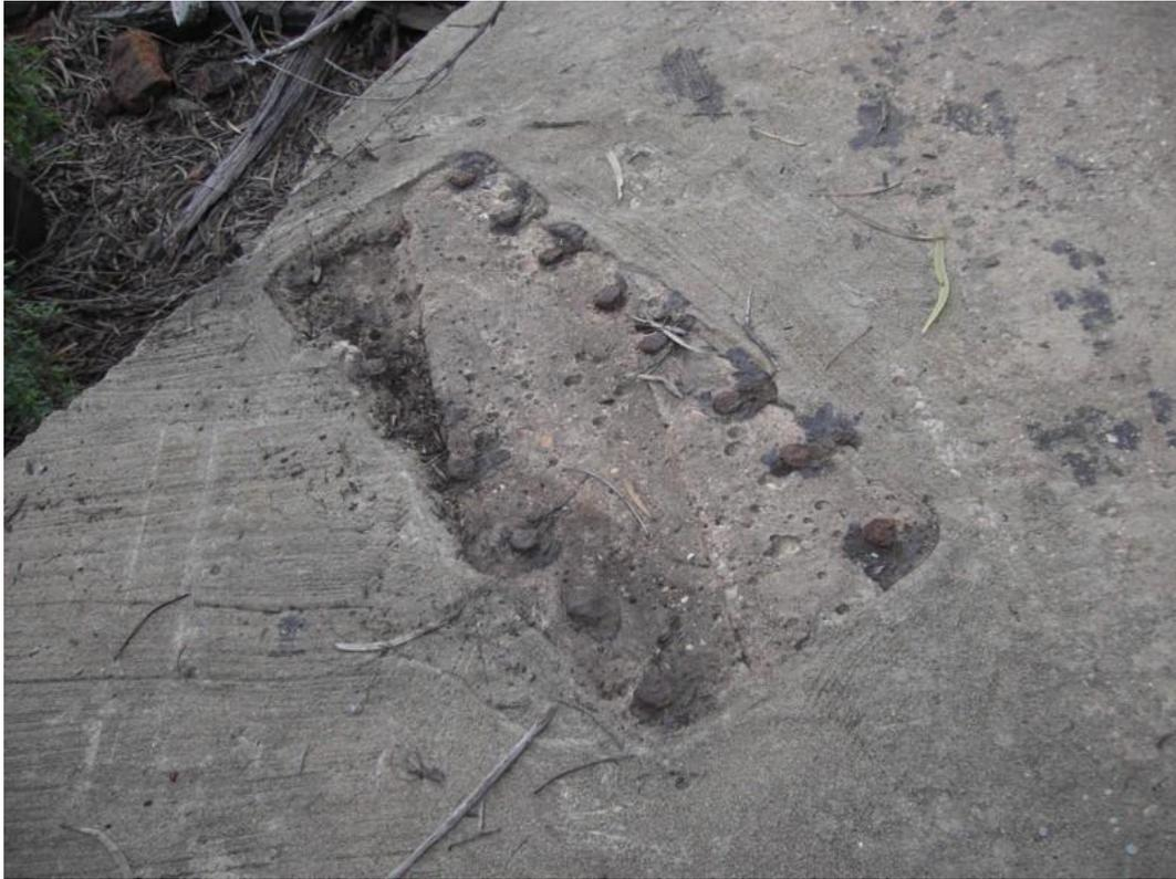
*Photo 3: The 16 cut of bolts where the 4 accommodation cranks were bolted.*
