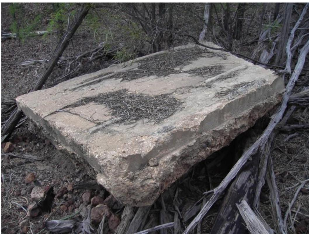
*Photo 1: The large piece of the concrete foundation showing the two ridges of concrete running lengthwise.*
